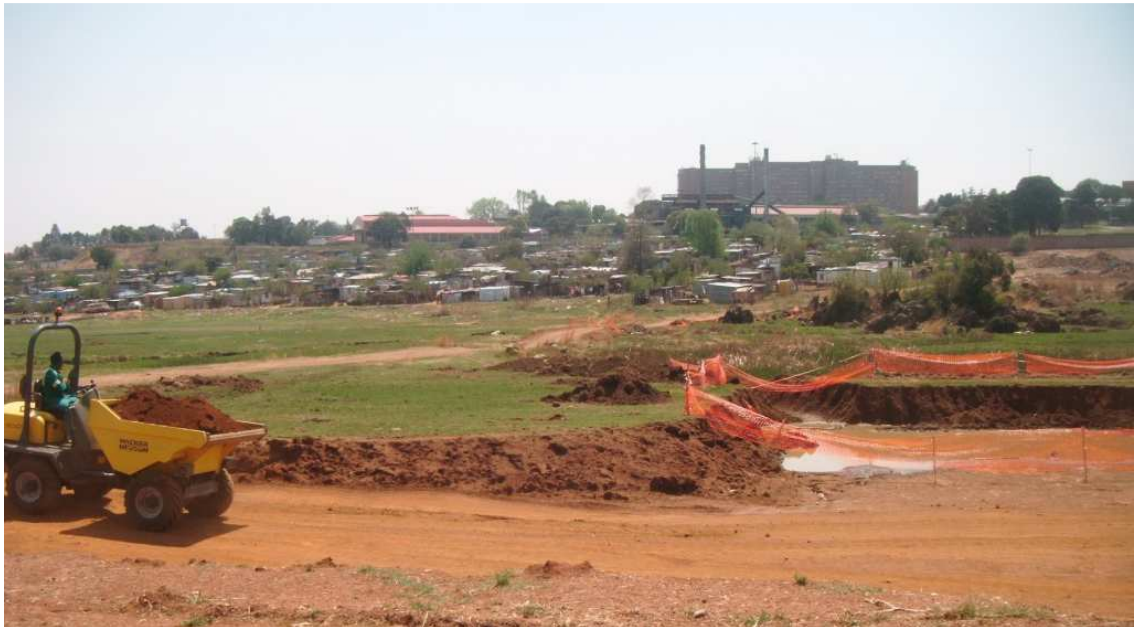
Figure 5.7 Ongoing construction activities on the Elias Motsoaledi Housing Project, with the settlement at the background. Source: Author's Photograph, September 2012.
