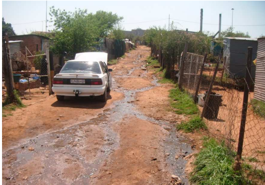
Figure 5.6 One of the roads opened up in the settlement showing the gullies that convey runoff.
