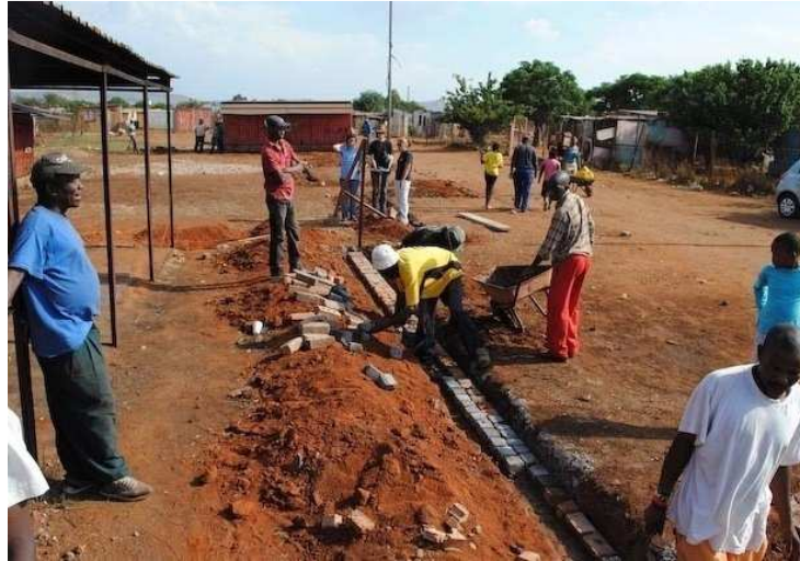
Figure 6.10b University of Pretoria Students and Community members constructing the Slovo Park Community Hall.
