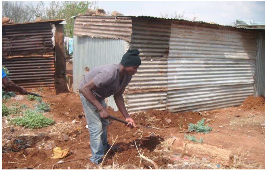
Figure 6.3 Heaping sand to the wall base for increased stability and barrier against runoff
