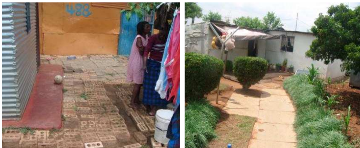
Figure 5.12. Other kinds of Stormwater Management strategies in Elias Motsoaledi. Paving made from perforated brick to aid permeation of runoff (left). Vegetation/Green Infrastructure in one of the stands (right). Not so widespread.
