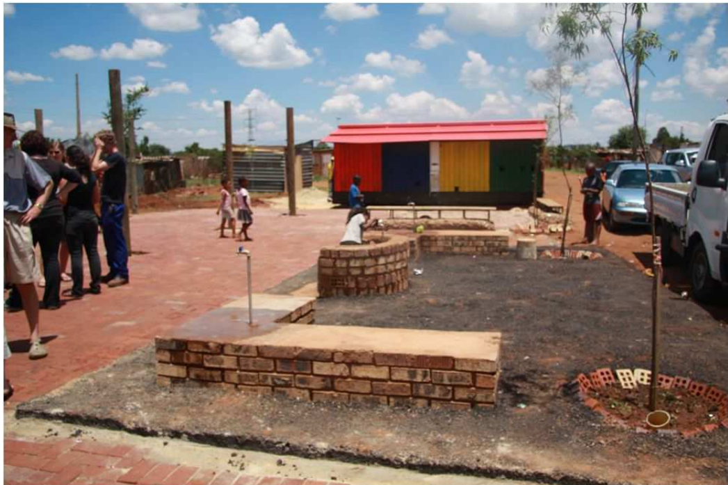
Figure 6.13 Taps and Trees, with the failed drainage system in the public space. Source: UP Slovo Park crew, 2010 (with permission).
