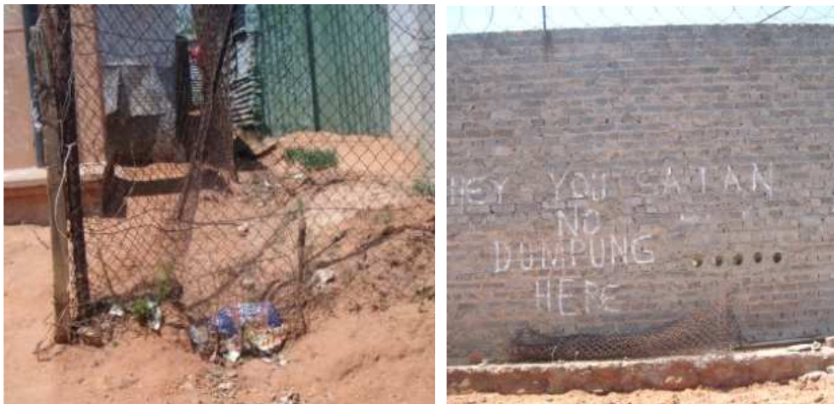
Figure 5.11 Stormwater Management strategies in Elias Motsoaledi. Waste trap to keep runoff and the gullies free of rubbish (left). Wall notice warns against refuse dumping (right). Outlets on the perimeter wall discharge runoff from the adjoining Chris Baragwanath Hospital.
