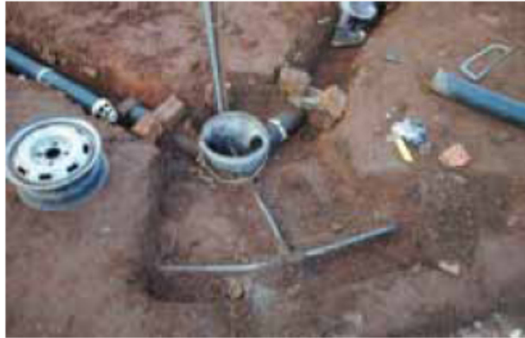
Figure 6.12 Drainage System in the Community Hall precinct under construction Source: Slovo Team, 2010 (with permission).
