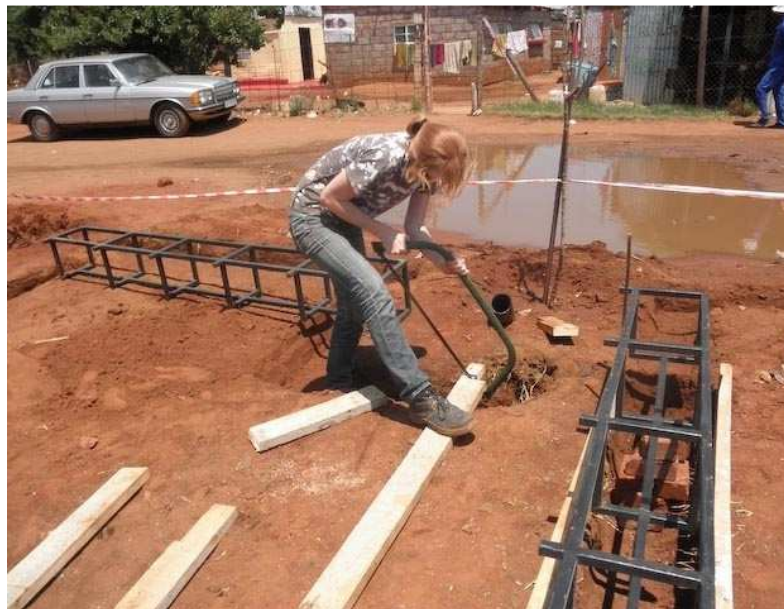
Figure 6.10a University of Pretoria Students and Community members constructing the Slovo Park Community Hall. Source: UP Slovo Park crew, 2010 (with permission).
