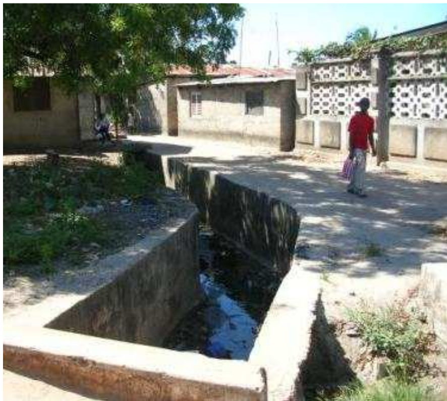
Figure 4.2. One of the completed drains in the Hanna Nassif settlement.
