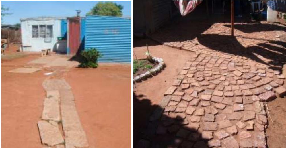
Figure 6.4 Walkway paving within stands. Source: Author's Photograph, September 2012.
