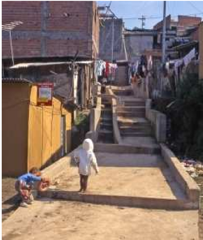
Figure 4.3 Stormwater drain and walkway constructed through the slope in Guarapiranga settlement
