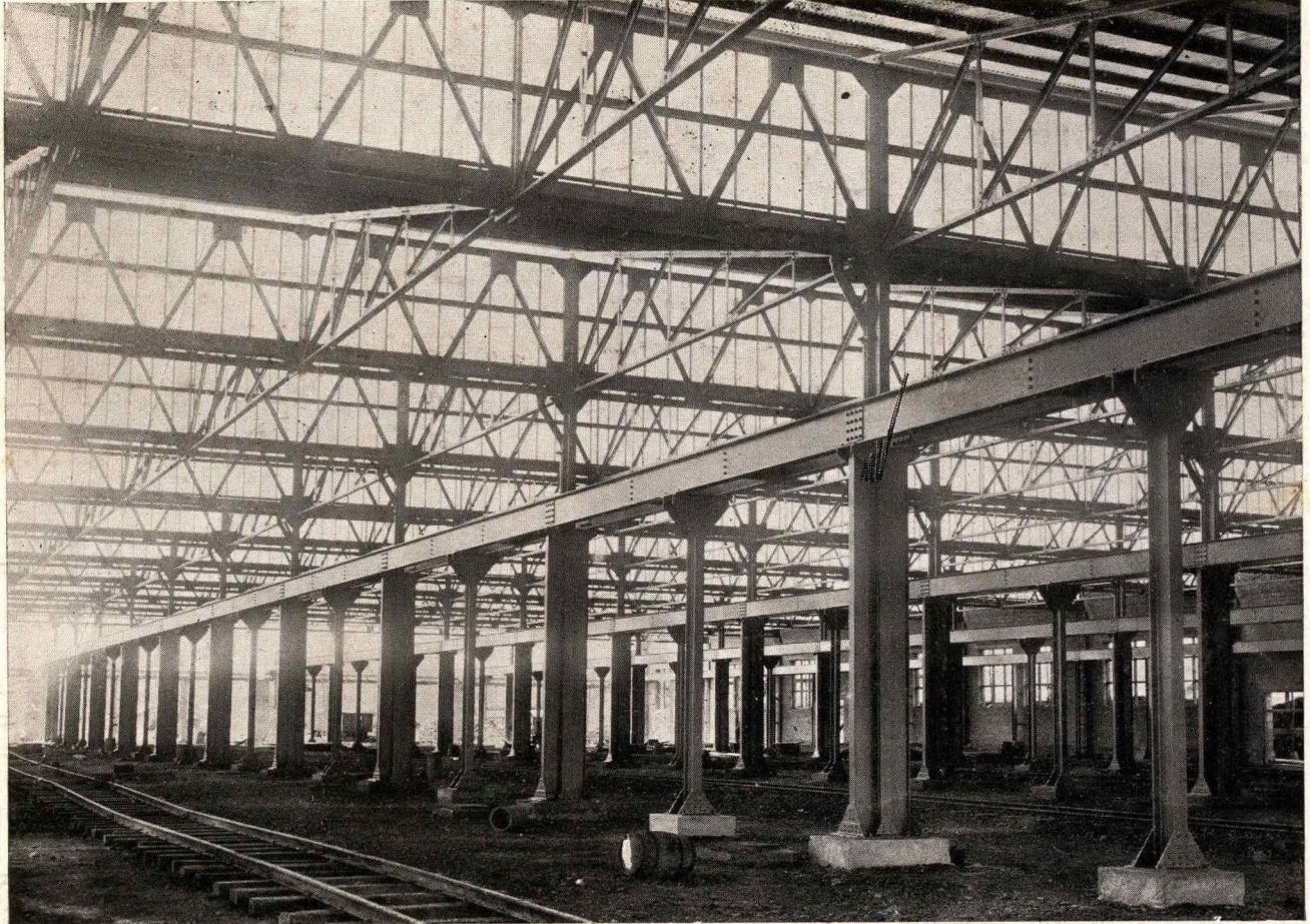
Internal View New Waggon Shops, S.A.R., Maritzburg. Total Weight of Structural Steelwork, nearly 1,000 tons. Supplied and erected by us complete.
