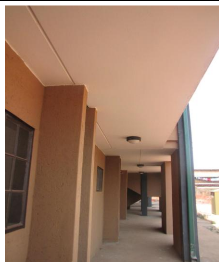
Ground floor view
