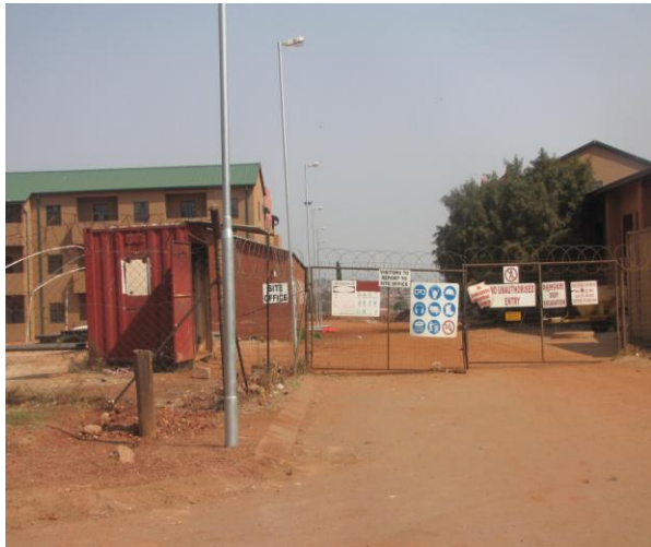
The entrance into the construction site of the family units and the site office which is situated within the vicinity of the site.
