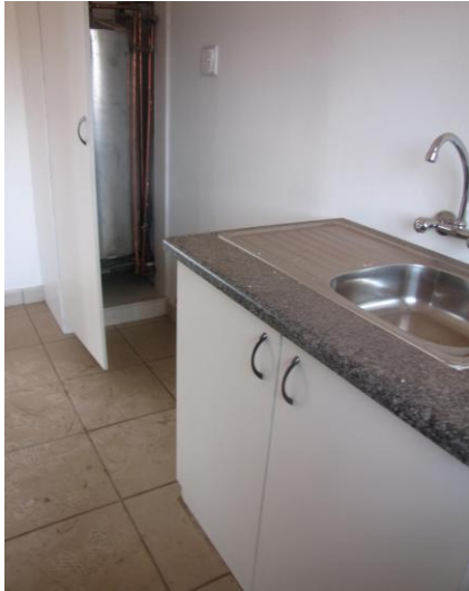
Built-in sink and geyser.
