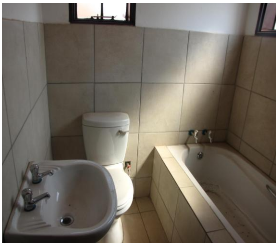
Each unit has its bathroom with a built-in toilet, bath and shower.
