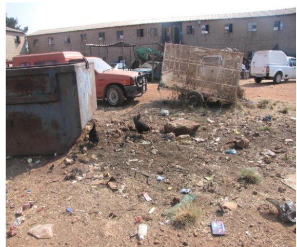
The hostel is in an obvious state of neglect and refuse removal is ignored.
