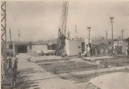
The kitchen and bathroom section is swung into place on the foundation. A plumber is connecting kitchen installations. The front lawn has been dug up and some shrubs planted. Other shrubs (far right) are ready to be transplanted to the grounds by a landscape gardener working with the construction crew.
