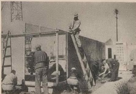
The main wall, with door attached, is fastened to the foundation by workmen. The bedroom (right) is in place and the furniture has been moved in. Through the window (center) a man may be seen laying the living room rug. At right, gardeners continue work on the grounds.
