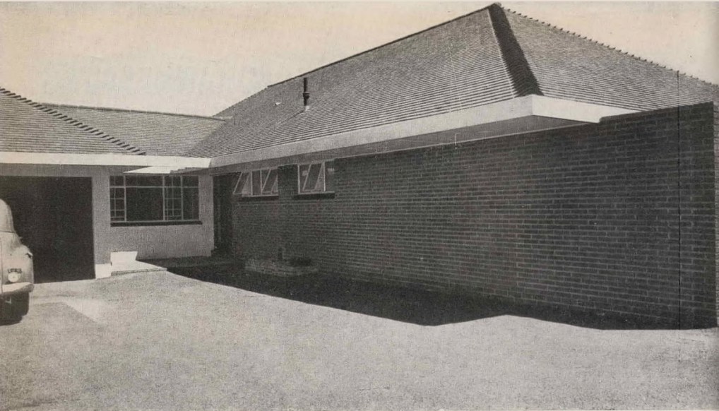
View from drive looking towards entrance.
