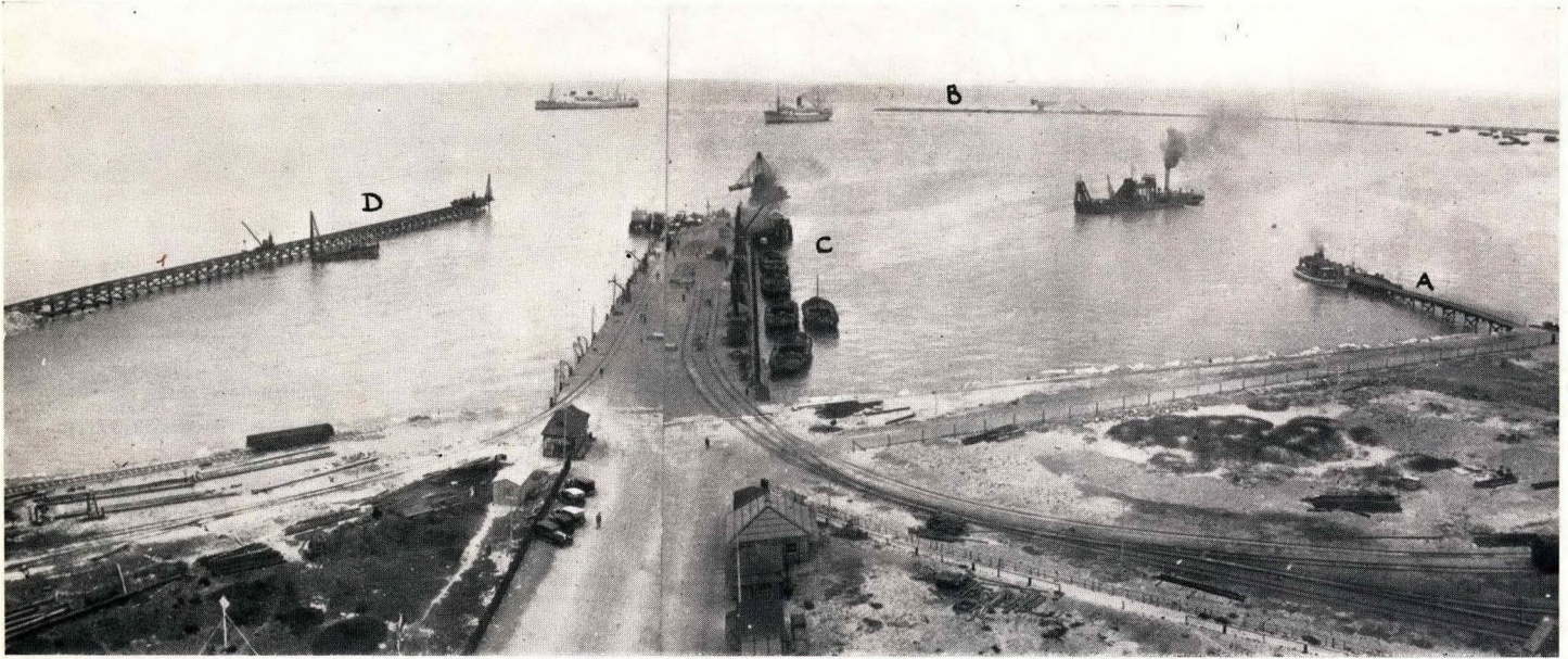
A Temporary Passenger Jetty. B Breakwater now Completed. C Existing Passenger Jetty now Closed. D Preliminary work in connection with North Arm of Docks. Note. —The whole area of foreshore shown in this photograph is reclaimed ground.
