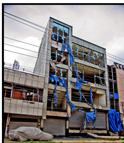
Figure 2: Sealed Building on Mehrauli-Gurgaon Road, sealed in 2006 15
