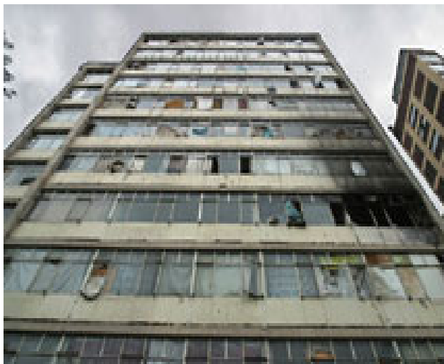
Figure 4: San Jose Building circa 2004 22
