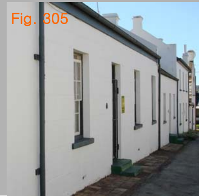
D. Houses in the colonial part of town built right on the Erf boundary, with less than a meter side-walk and then the street. (Fig.305)
