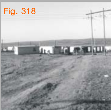
D. RDP houses in extension 8, built after 1994.(fig318)
