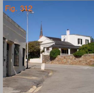
K. Artisan square. Houses on intersection respecting a 45 degree angle on the corners, creating a square in a residential minor road.
