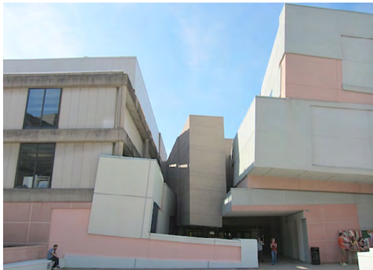
Figure 48: The main entrance to the Aronoff Center. The new extension is to the right and the existing building is to the left of the photo. ( http://chronicle.com/blogs/buildings/files/2010/10/ )
