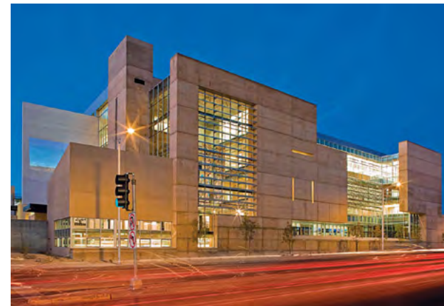
Figure 28 (top): Media screen (far left) and expanses of glazing on Antoine Predock's (2009) School of Architecture.
