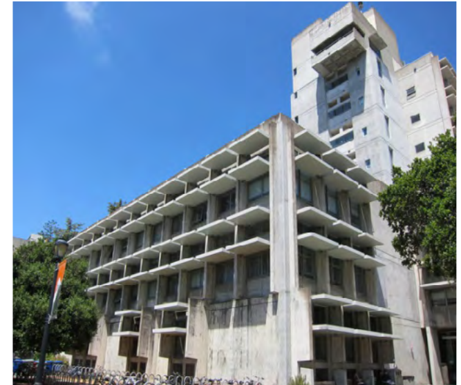
Figure 27b (below): Wilkinson building, Sydney University School of Architecture ( www.sydneyarchitecture.com/UNI/UNI-069.htm )
