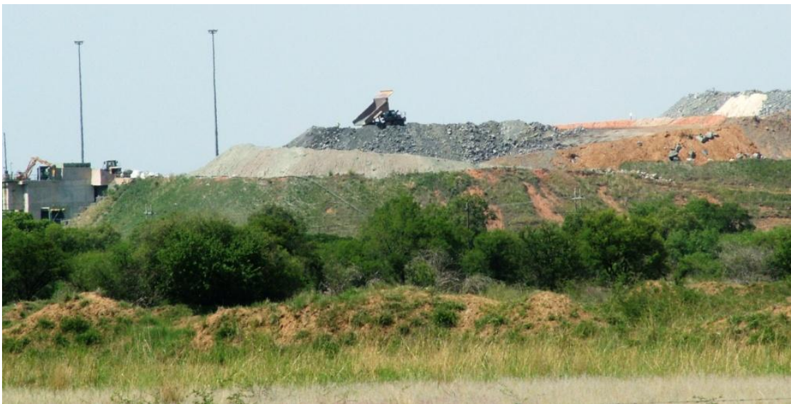
Figure 12. Photograph of platinum tailings with a dump truck on top of a tailings dump [Aquarius platinum mine] (G Nelson)
