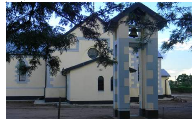
Fig 6.15. The bell tower on the eastern end of the site.
