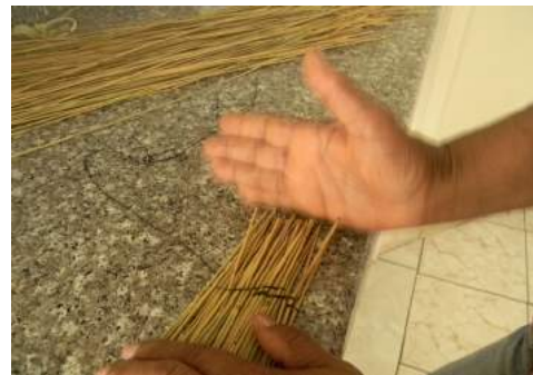
Adjusting the edges of the thatch.
