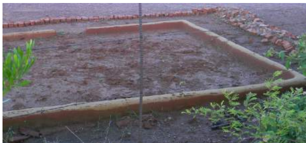
Fig 5.16. An example of the foundations of a traditional Setswana home
