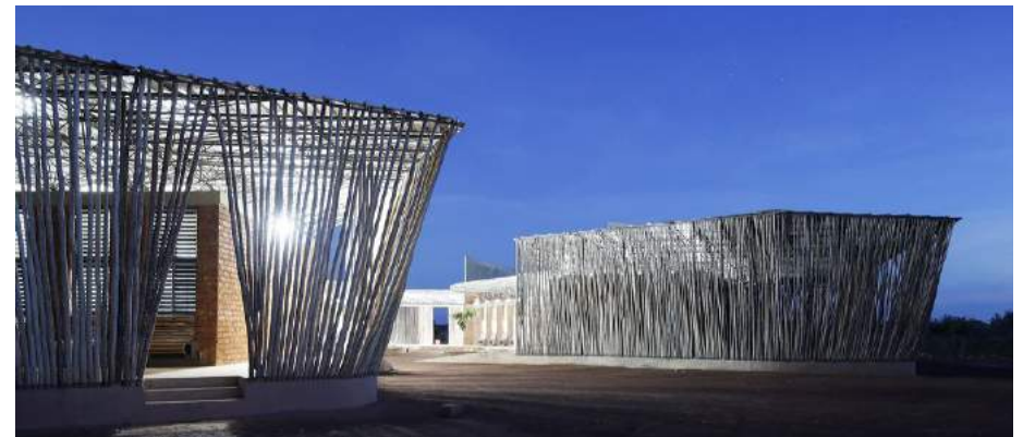
The layered facade of the school
