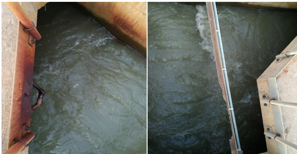
Figure 1.2: Coagulation unit where \text{FeCl}_3 and polyelectrolyte are dosed
