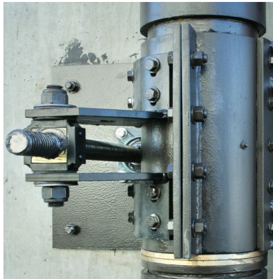
Fig 6.3- Art Stable Joint detail
