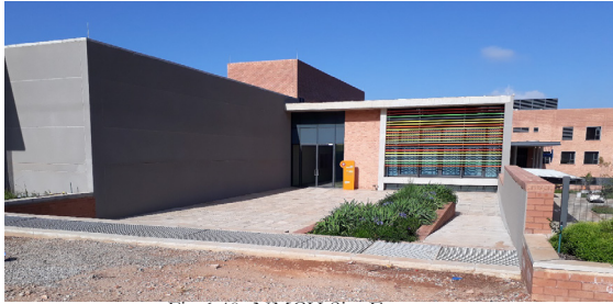
Fig 6.40- NMCH Site Entrance
