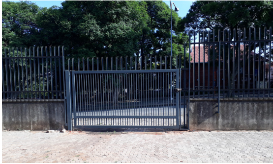
South Gate entry onto Jubilee road
