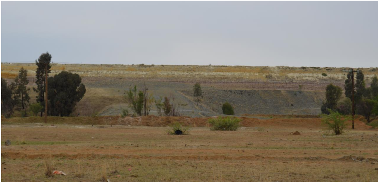
Figure 54. The repaired section of wall of Merriespruit No. 4 tailings storage facility in October 2015 (Source: Author)
