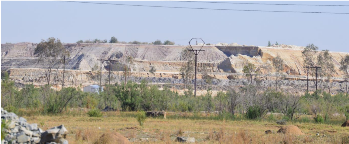
Figure 80. View of re-mining of the Harmony north tailings storage facility, October 2016 (Source: Author)
