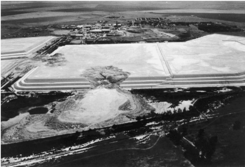
Figure 52. The tailings failures at Saaiplaas tailings dam in March 1992 (Fourie et al., 2001)
