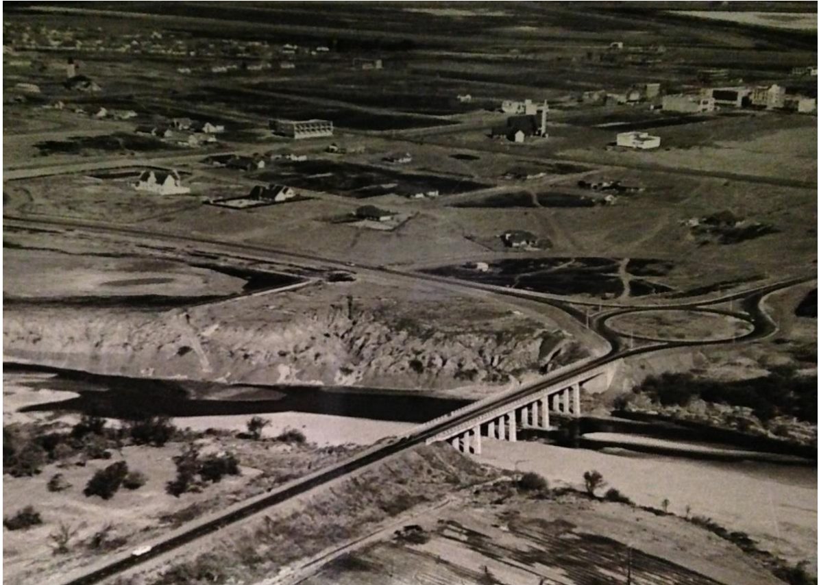
Figure 23. The growing town of Virginia around 1955, showing the newly constructed Voortrekker bridge over the Sand River (Source: Welkom Public Library)
