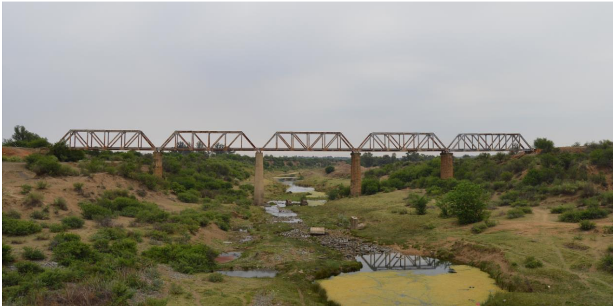
Figure 13. The original railway bridge across the Sand River in October 2015. The second support was repaired having been blown up in 1900 (Source: Author)
