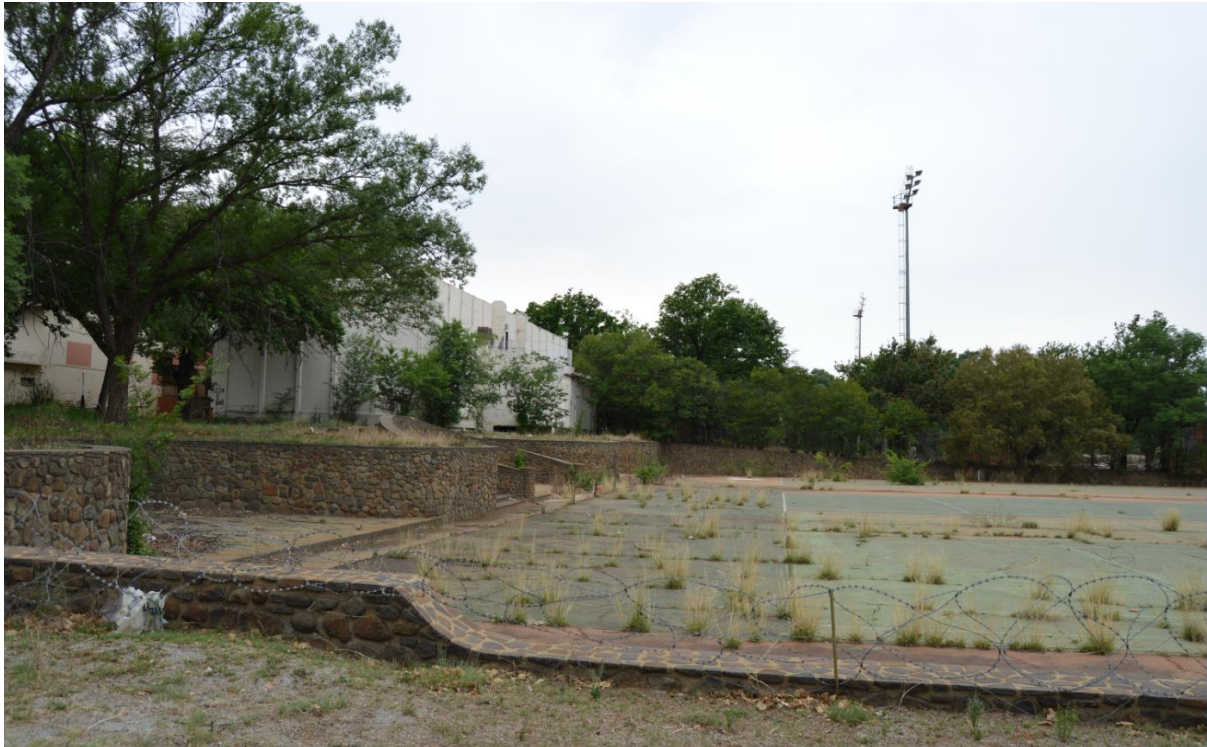
Figure 84. The abandoned Harmony Country Club, October 2015 (Source: Author)
