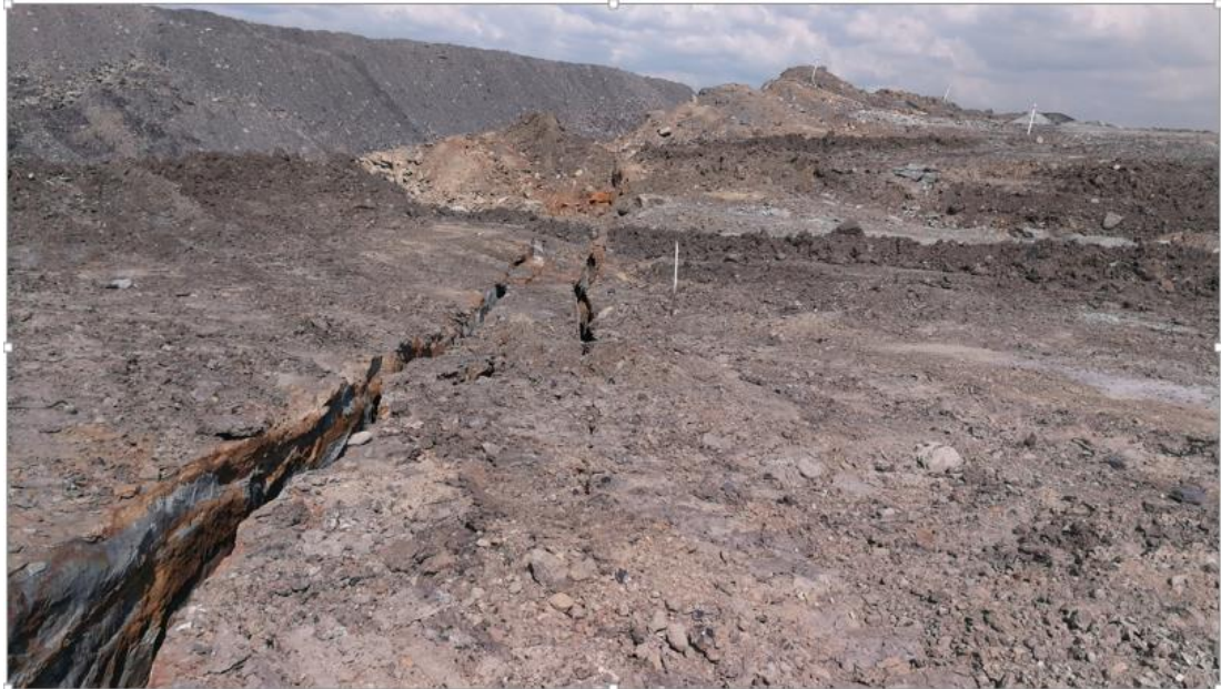
Figure 4.3.4 Blast induced cracks sympathetic to dyke 1 in Strip 31 North Pit
