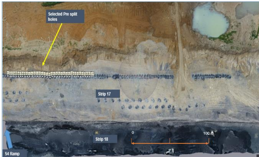
Figure 4.4.2 Pre-split holes in Strip17
