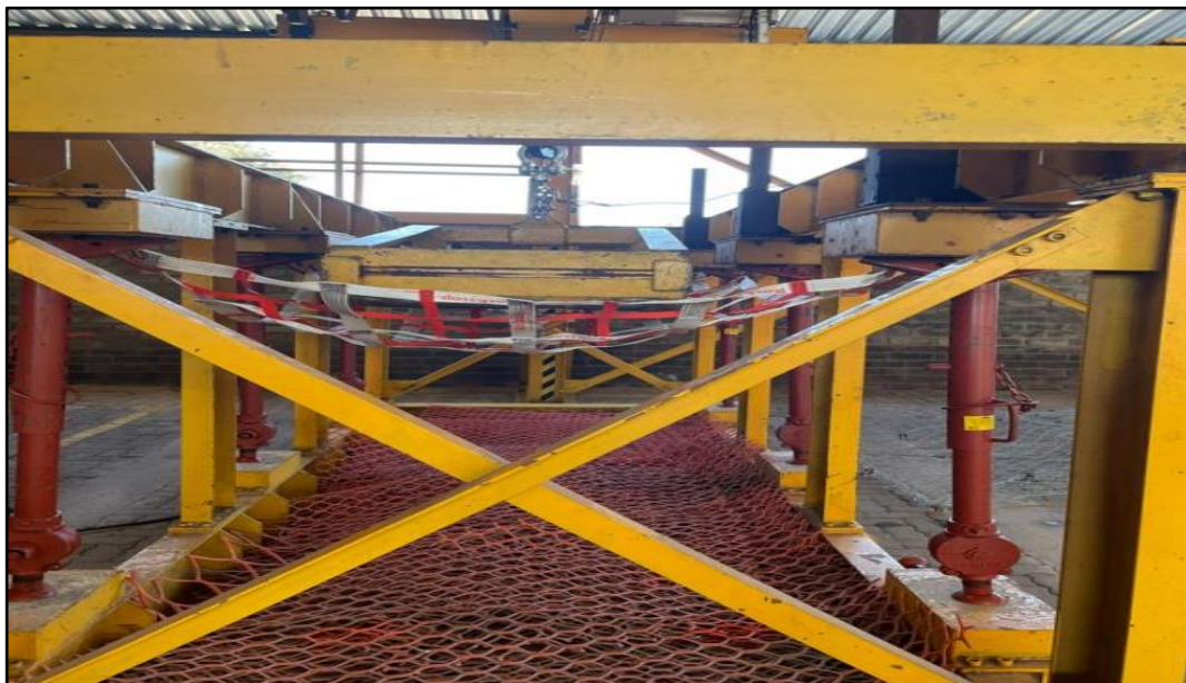
Figure 3-4: NCM Frame 2 for testing of mechanical props with safety nets
