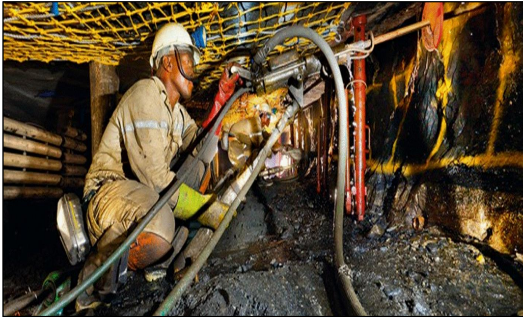
Figure 1-7: Typical temporary support on a stope panel face area (Mutsvanga, 2018)
