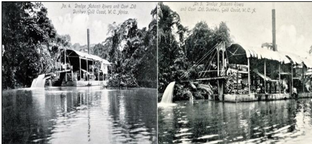
Figure 5.4: Dredgers mining gold in Dunkwa in 1910. Source: Mindat.org (1985)
