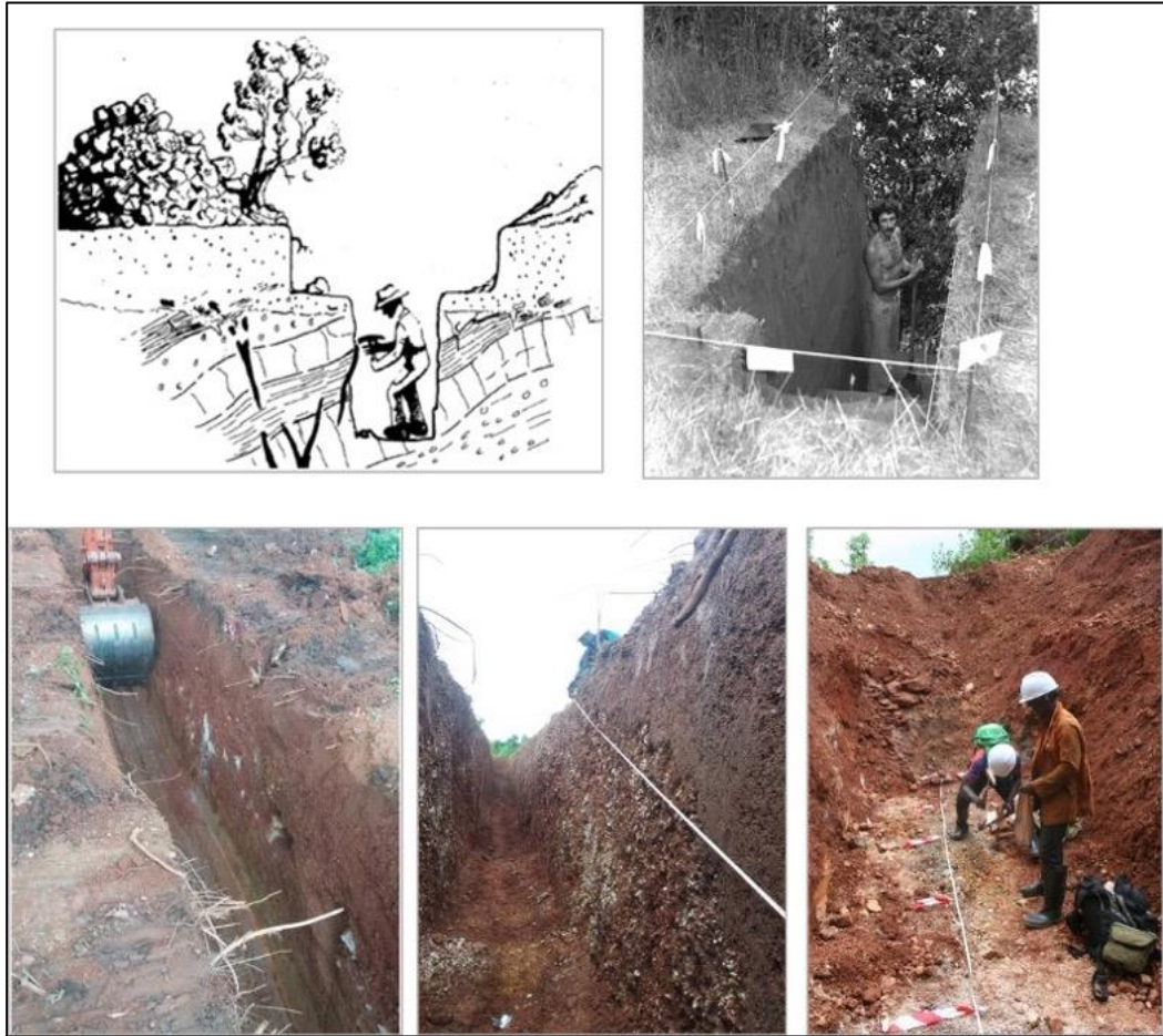
Figure 4.5: Trenching exploration method. Sources: Force Commodities (2018); CSE Landscape Architect (2012); Geology Hub (2017).
