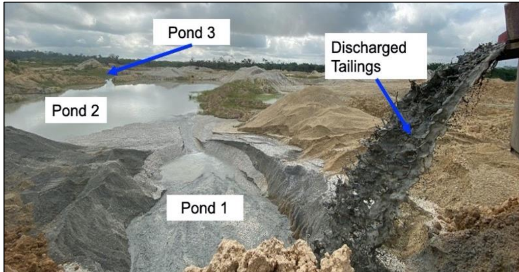
Figure 5.20: The 3-pond water purification system on the mine
