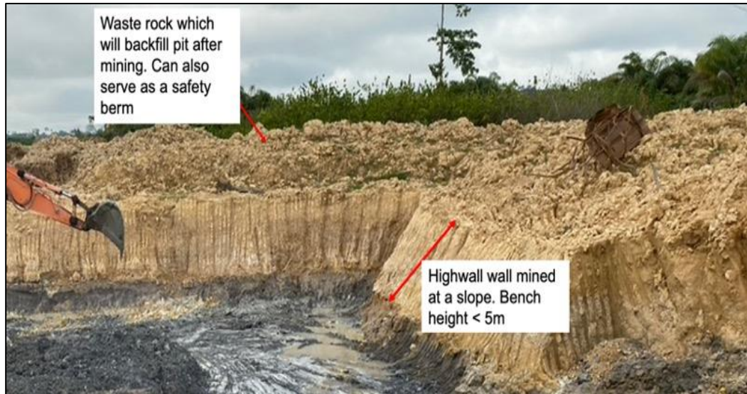
Figure 5.16: Geotechnical engineering principles observed on one of the legal mines
