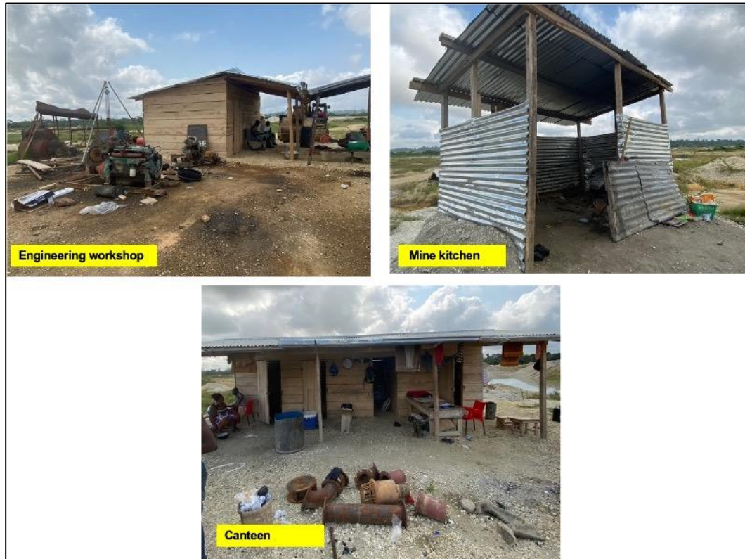
Figure 5.12: Camp facilities observed on legal mines
