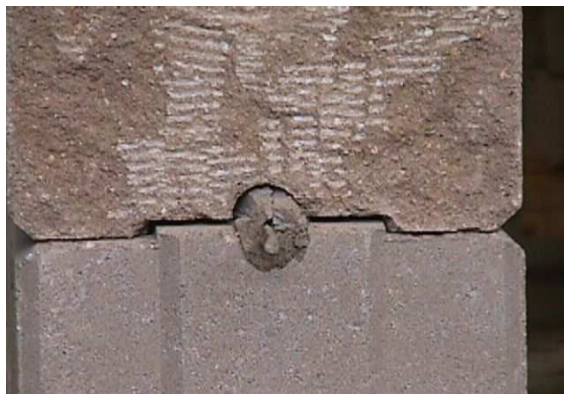
Figure - 5.5: Dry-stack feature and reinforcement detail
