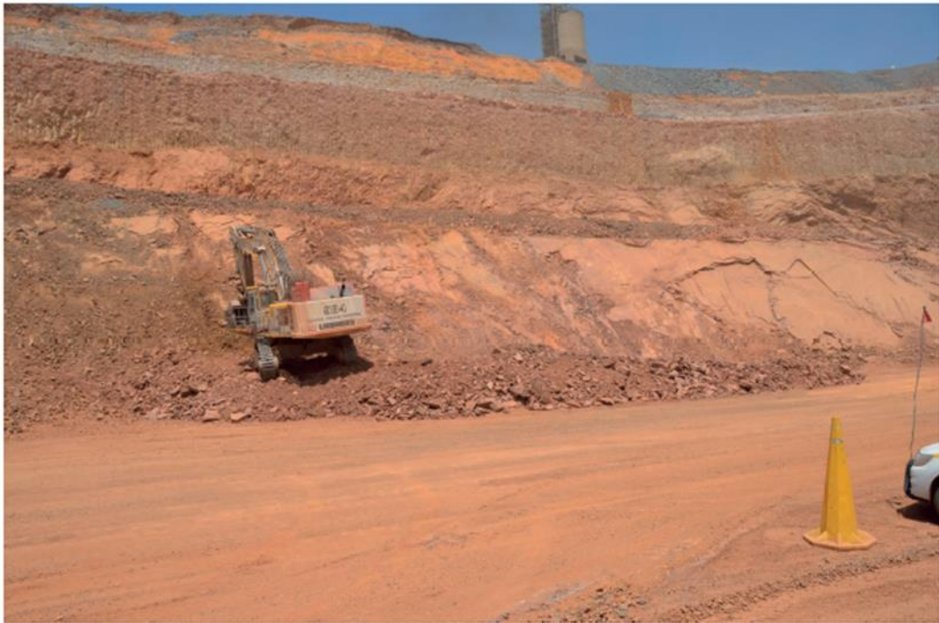
Figure 119 An excavator scaling and loading a final pit boundary ( Gabanakgosi, et al., 2018 ).
