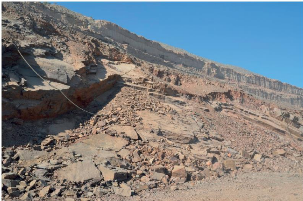
Figure 116 Planar type bench failures at Jwaneng Mine Cut 8.
