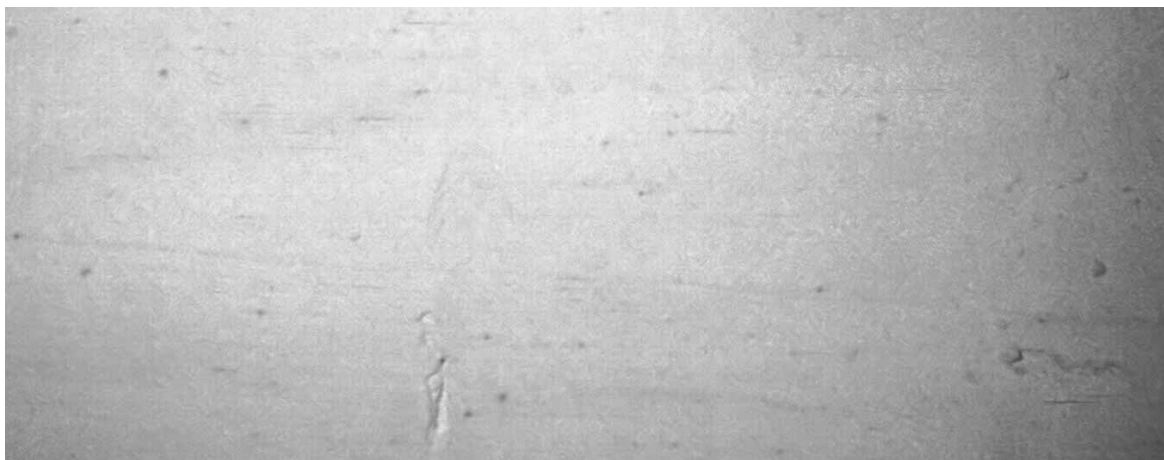
FIGURE 28: Specimens coated with cementitious based coating
