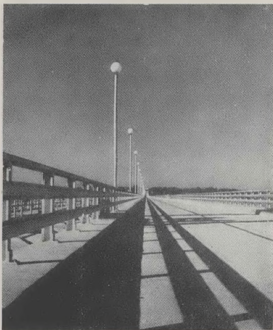
The Roadway over the Wheeler Dam displays a marked economy of form and material—simple light standards and railings of standard steel shapes.
