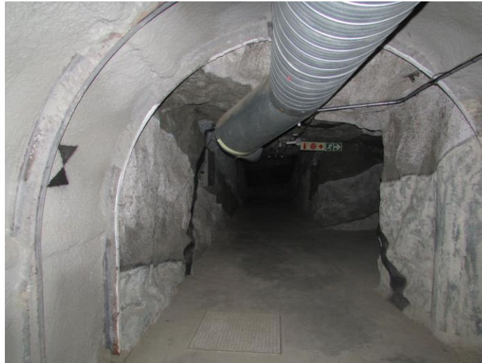
Figure 1-2 Nick's Tunnel showing steel arches, shotcrete, ventilation duct and stope breakaway
