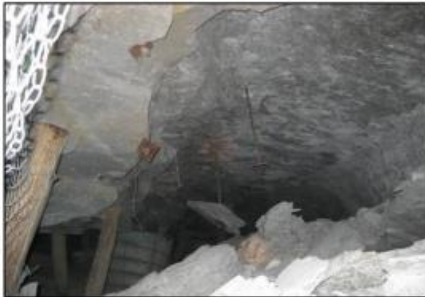
Figure 2-7 Fracturing of exposed rock in the Bushveld Complex (Mine Health and Safety Council, 2016)
