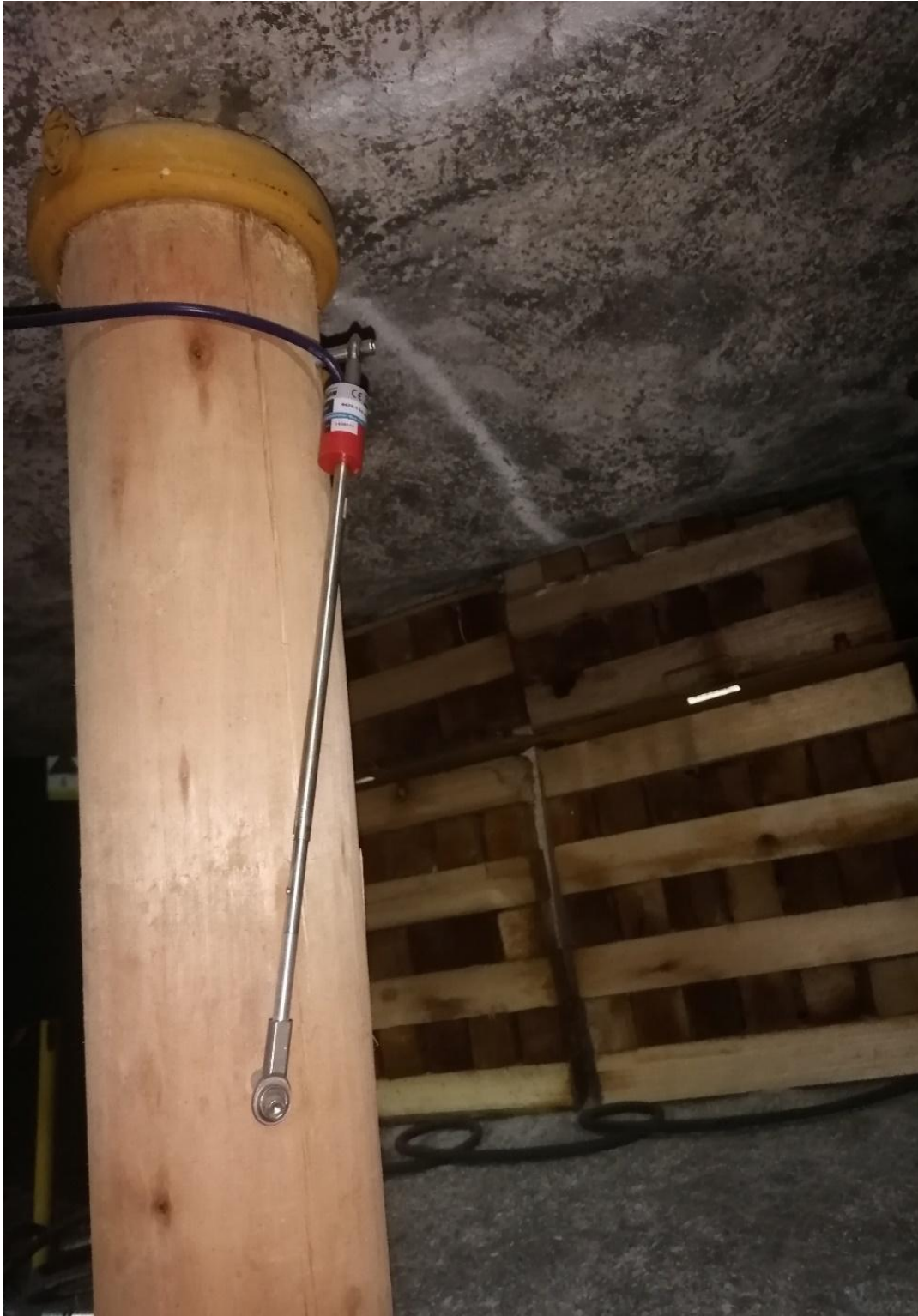
Figure 11: Strain gauge installed on the stope support.
