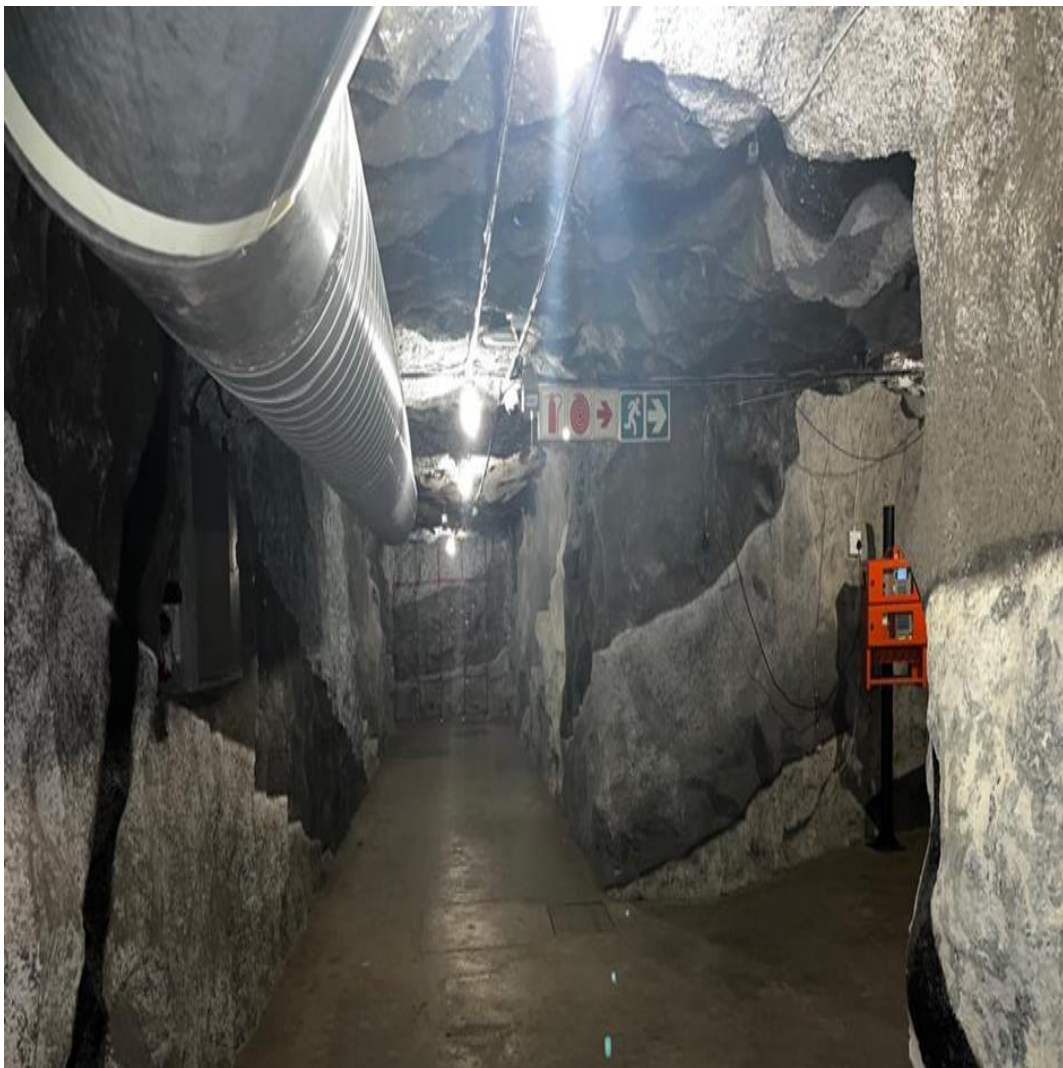
Figure 9: View Inside the Tunnel
