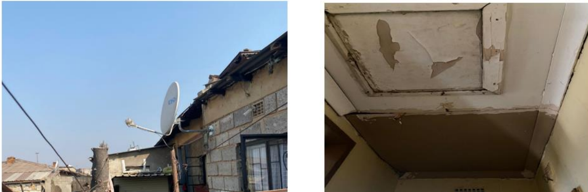
Figure 30. Exterior and interior views of the host household's roof.
