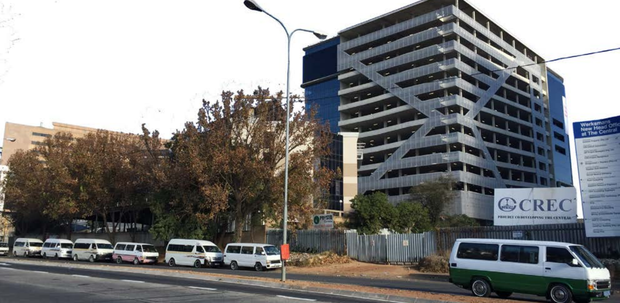
figure 4,8. Taxi waiting outside of a construction site on Katherine Street
