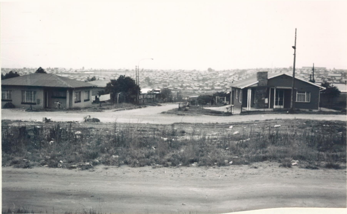
Fig 3.3 Houses in Soweto
