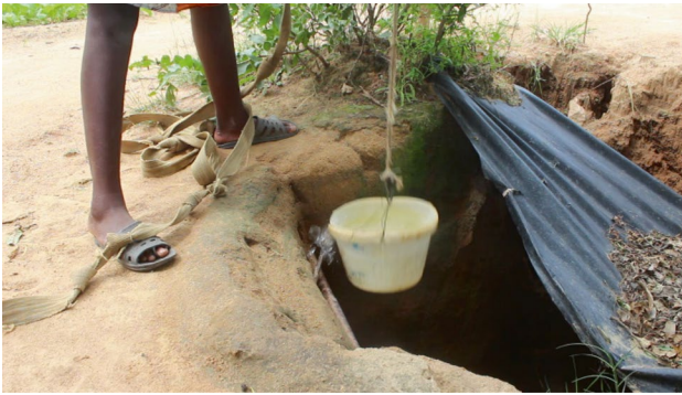
Fig. 4 A dugout well. Source: Authors' fieldwork
