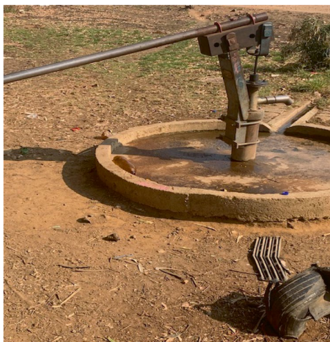
Fig. 5 A typical borehole (bush pump) in Zimbabwe. Source: Authors' fieldwork
