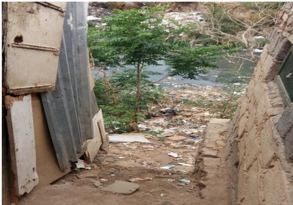
Fig 4.2 Structures located in the flood plains of the Jukskei River in Stjwetla Informal Settlement Source: Own (2019).
