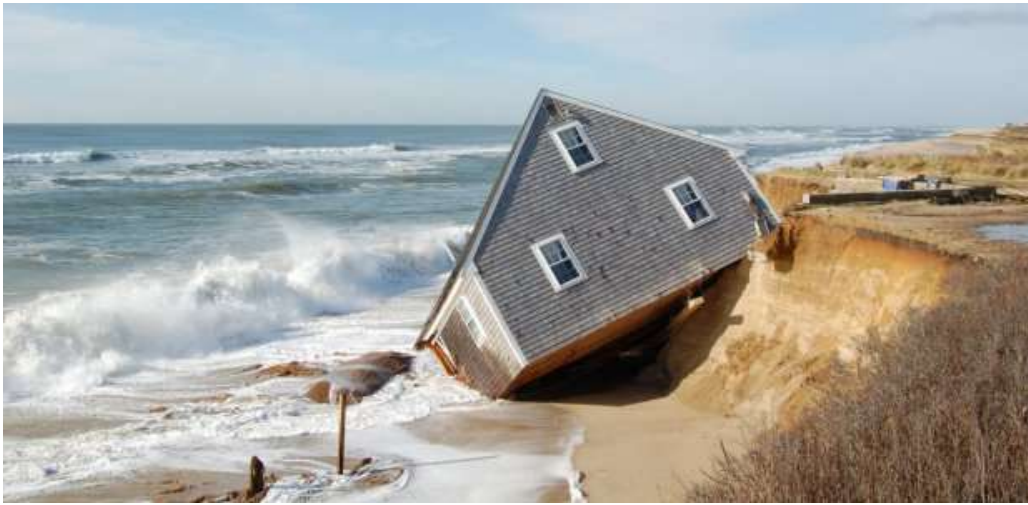
Figure 4: A house in Sheep Pond Road Madaket Massachusetts (USA) collapsed due to beach erosion (Brace, 2015)
