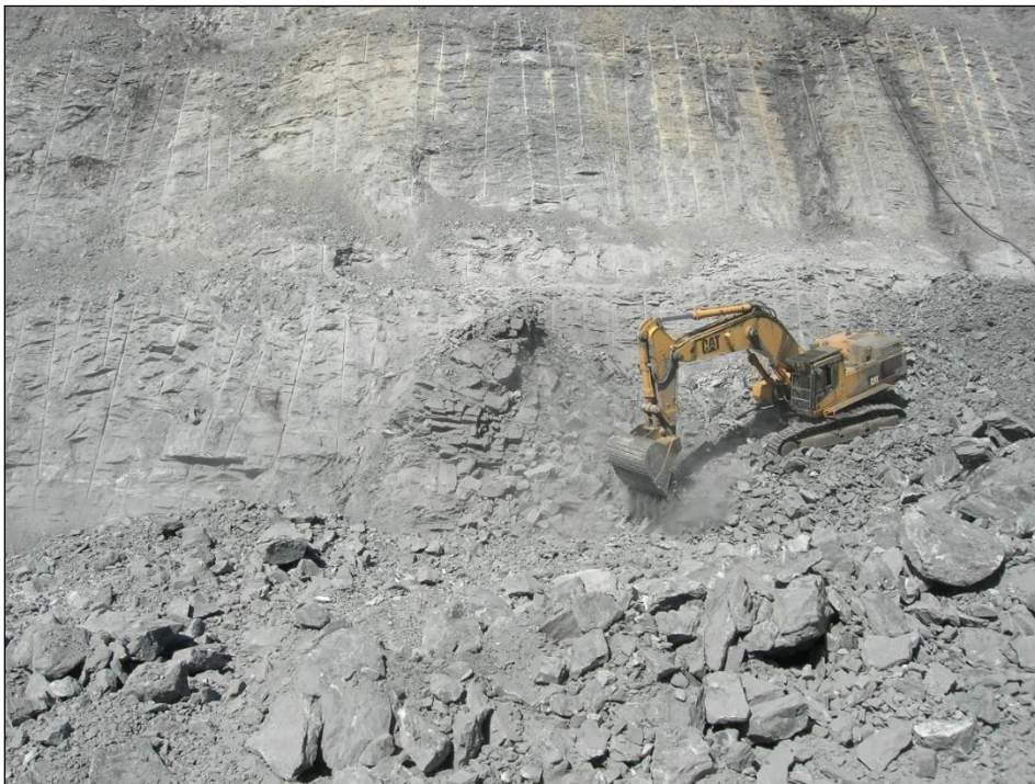
Figure 4.1: Evidence of pre-split blasting on Eastern side wall
