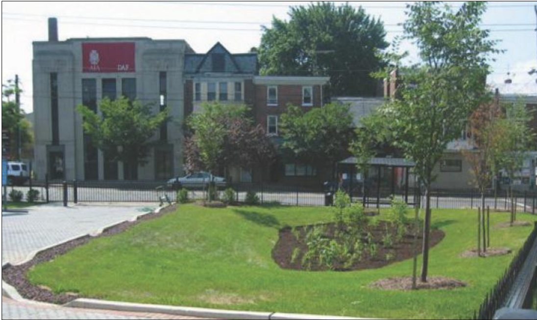
Figure 11: Green infrastructure design principles in Wilmington, Delaware designed to absorb and retain storm-water runoff (EPA, 2008).
