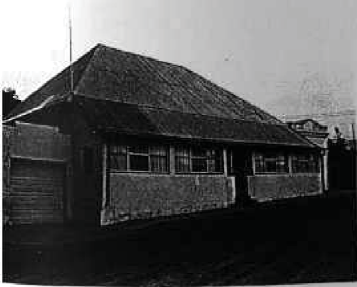
Erf 210: 7 Murray Street. (Street converted Rissolier Canyon).
