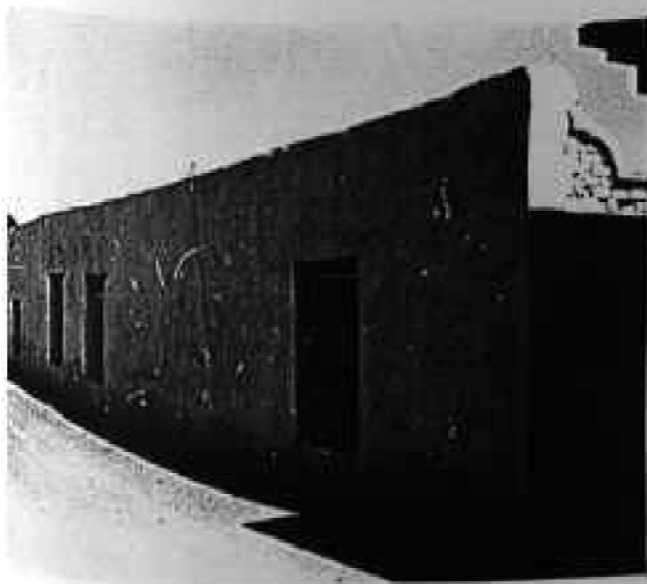
ven 195, 196 & 197: Side facade of 27 Murray Street.
