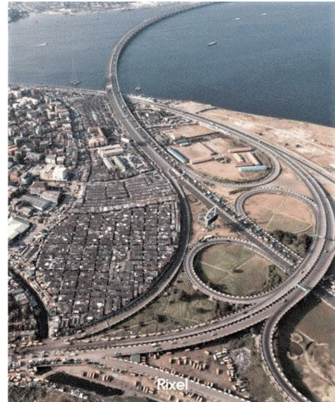
Photo 4.8: Picture showing parts of the 3 rd mainland bridge. (Source: courtesy of Auto Josh Blog, 2021)
