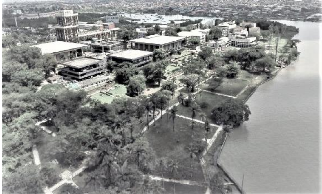
Photo 1.2: Aerial view of the first phase of the Unilag development overlooking the lagoon (Source: Info@lagosviews.com , accessed [2019])
