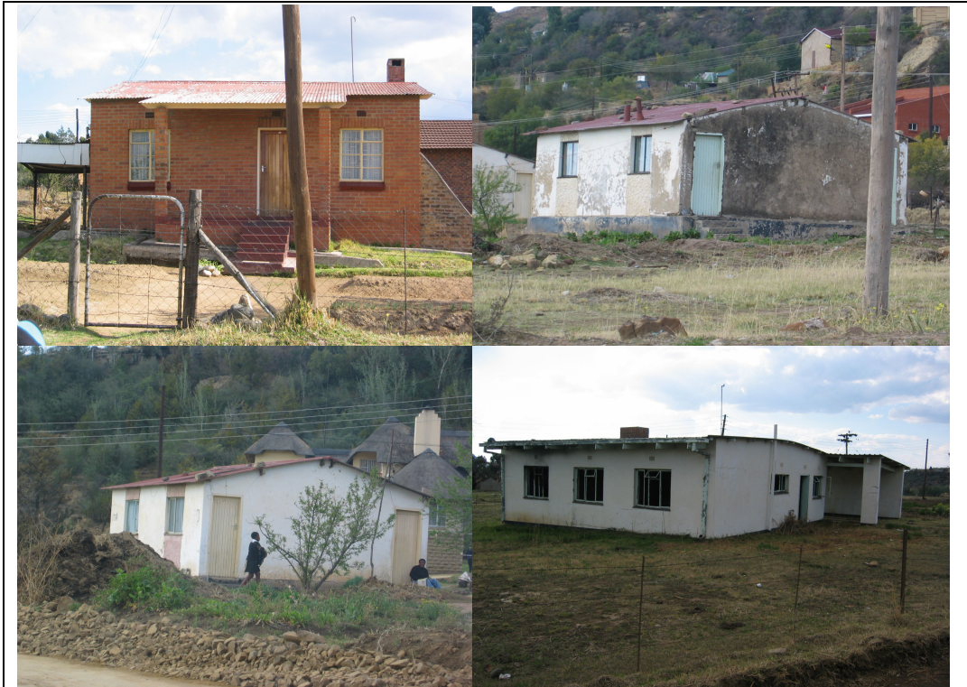
Figure 4.17 Govt housing structure
