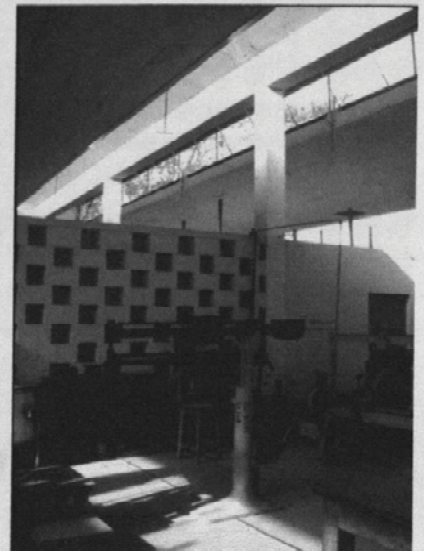
6.3 James Cubitt, interior of Engineering Block KNUST 1951 in 2001 (photo Hannah le Roux)
