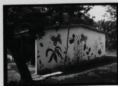
6.7 James Cubitt, Type 'B' house in 2001 (photo Hannah le Roux)
