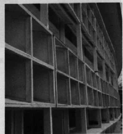
5.8 Fry, Drew and Partners Sunscreens at Prempeh College, Kumasi, Ghana 1955 (photo Hannah le Roux)
