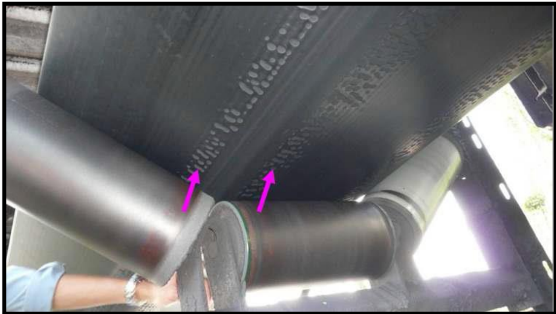
Figure 2-15: Damage on bottom cover due to high contact pressure (Zhang, 2015).
