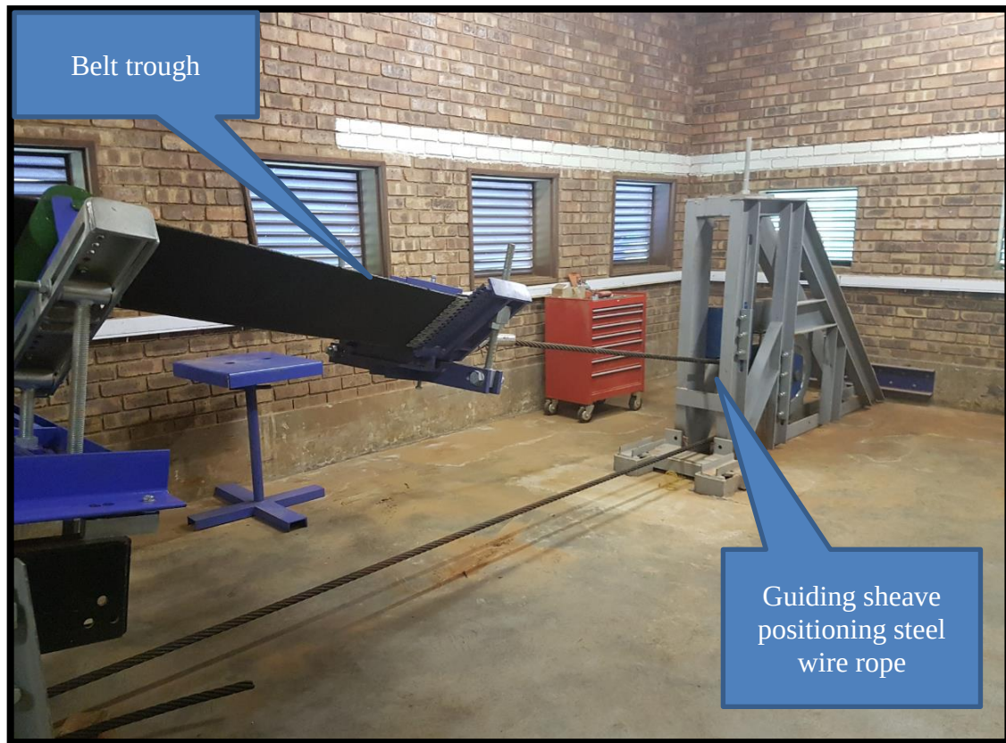
Figure 4-42: Guiding sheave directing the steel wire rope.
