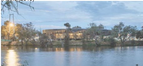
Fig 5.3 View of building from across river Avon (Archdaily, 2018)
