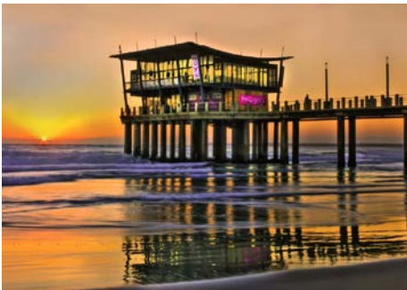
Fig 1.18 Photo of uShaka Pier, Moyo Restaurant(Moyo, 2019)
