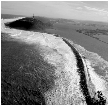
Fig 1.34 Durban South Pier, A photograph of the seas breaking the constraints of the pier during the Saros spring high tides, March 2007.
