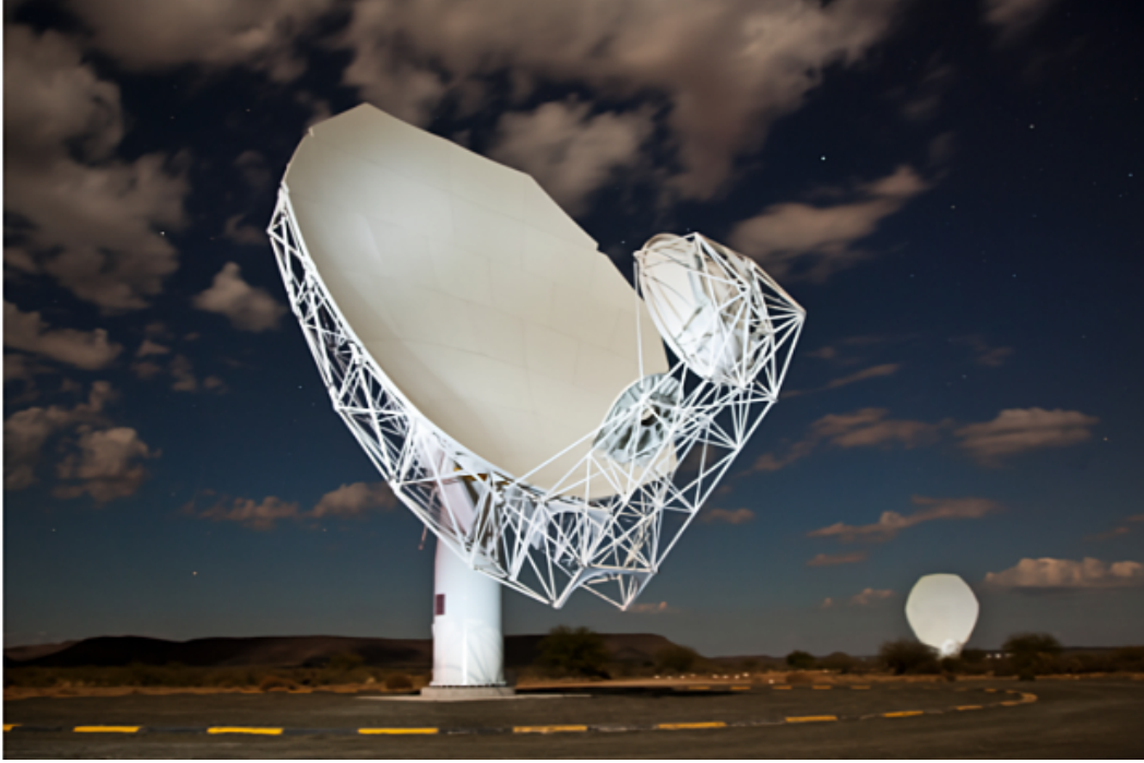
Figure 1.11: A MeerKAT antenna, with offset Gregorian feed. Source: [137]
