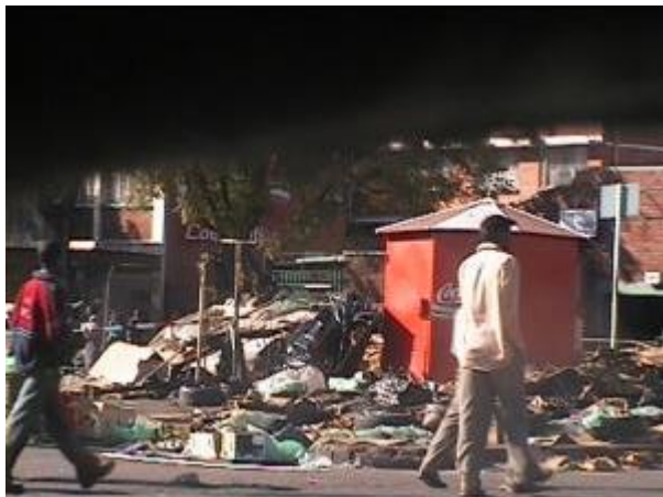
Figure 17. 3. Vendor's Market demolished
