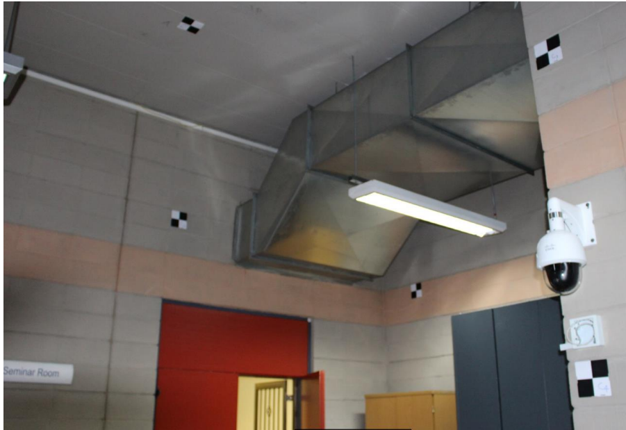
Figure 4.12: An Image Showing the Placement of Targets on the Concrete Wall and the Ceiling of the Scanning Laboratory
