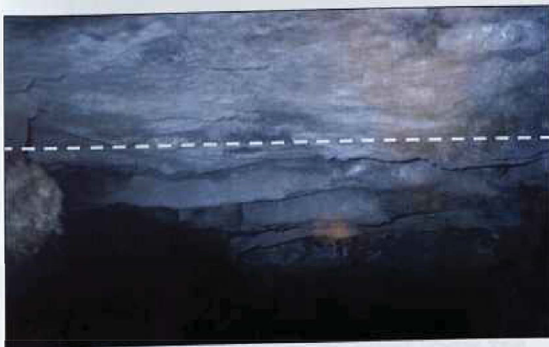
Figure 5.3.1 The improvement in hangingwall conditions brought about by the introduction of preconditioning
