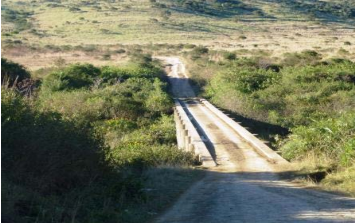
Figure 6. Gravel road with bridge (Source: Amajingqi Development Master Plan 2012)
