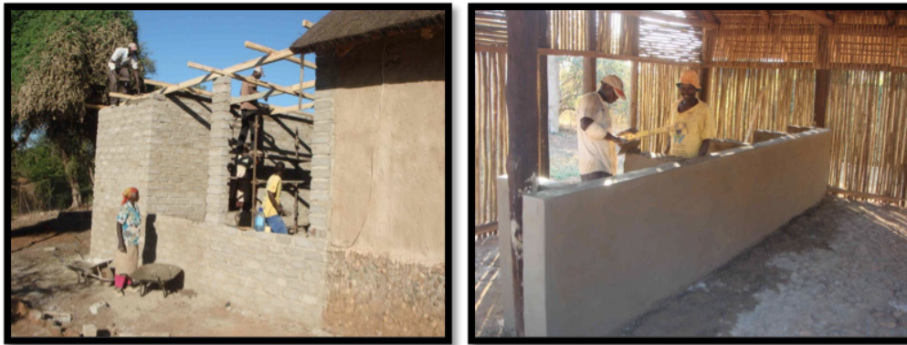
Figure 22 Makuleke B&B renovations in May 2008. (Photos: May Shehab 2008)
