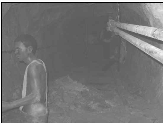
Figure 6- Digging in a new direction, setting up the framework Photograph taken by researcher
