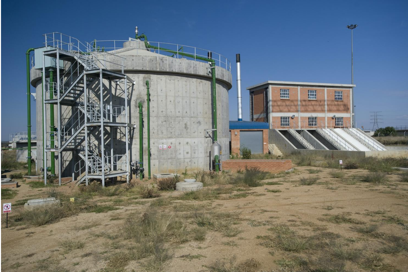
Grit Chamber - GWWP
