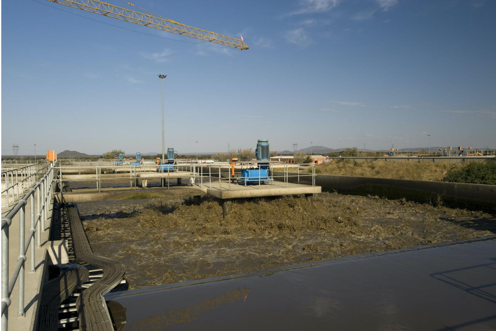
Sludge Pond - GWWP
