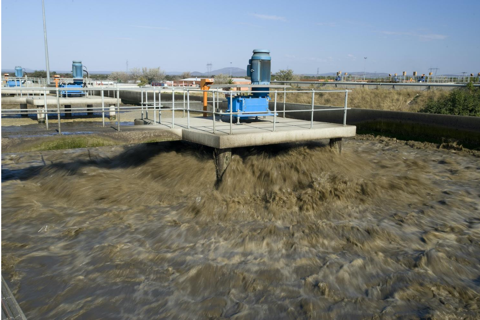
Sludge Pond - GWWP
