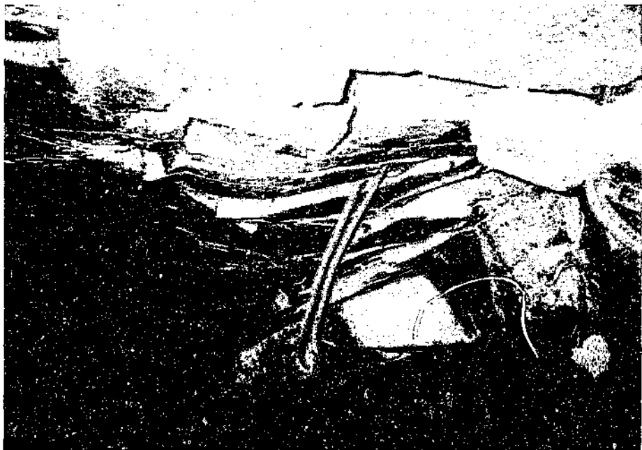
Plate 26 - Buckling Of The Hangingwall Over A Centre Gully.
