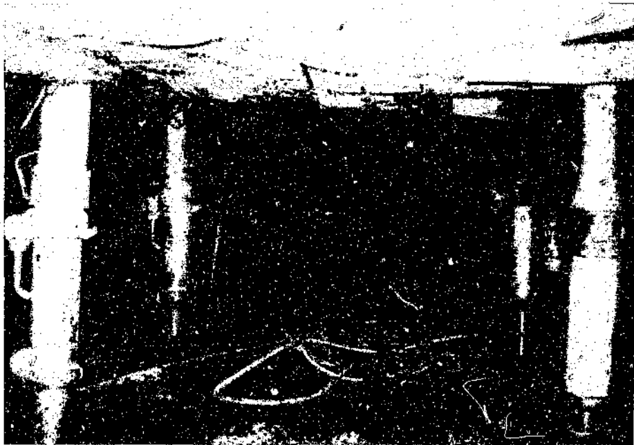
Plate 31 - Change-Over From 300kN Props To 200/400kN Props.
