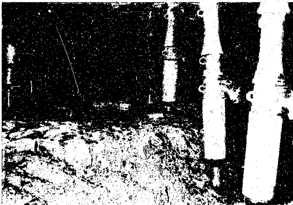
Plate 6 - 200/400kN Blast-On Props Installed In 78A-42W N7 Panel At No.5 Shaft.
