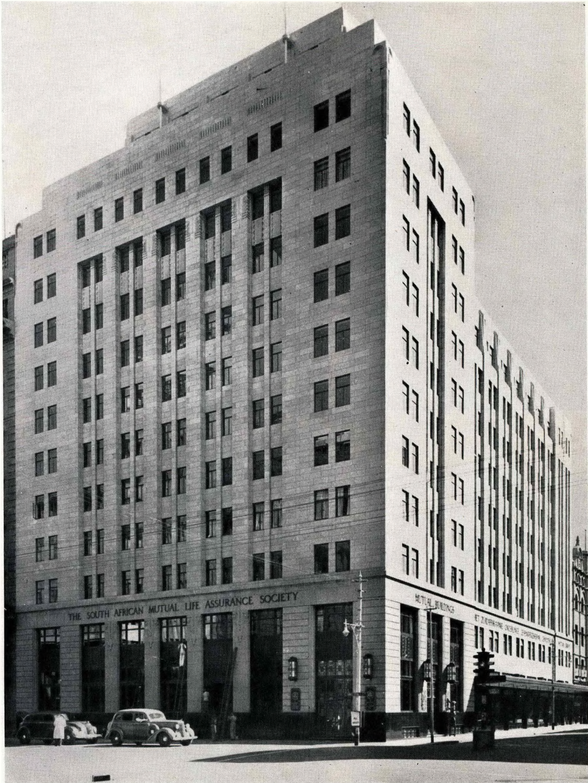
View from Corner of Harrison and Commissioner Streets Architects: Stucke, Harrison and Smail
