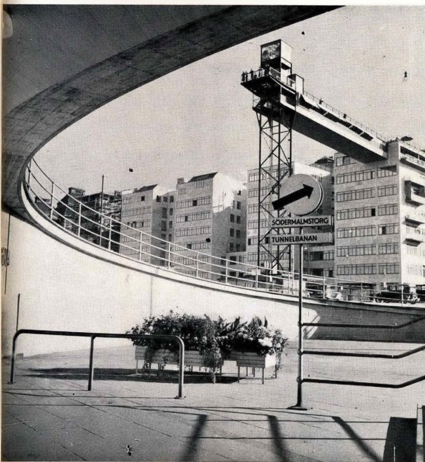
STOCKHOLM: The main office of the Co-operative Union as seen from one of the lower planes of the Slussen viaducts. The architect, Eskil Sundahl, has used marble for the surface of the walls. The connecting link between the building and the Katharina Lift houses a very popular restaurant, the Gondola.
