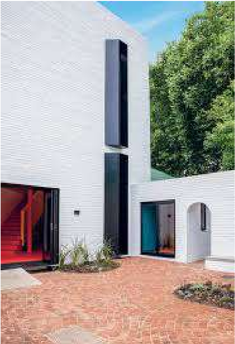
Figure 7.15: STEAM Centre (Meshworks Architects, n.d.)
