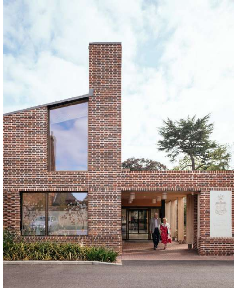
Figure 7.19: John Morden Centre (Mae Architects, n.d.)
