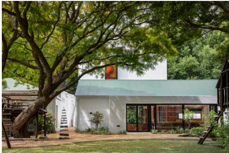
Figure 7.12: STEAM Centre (Meshworks Architects, n.d.)
