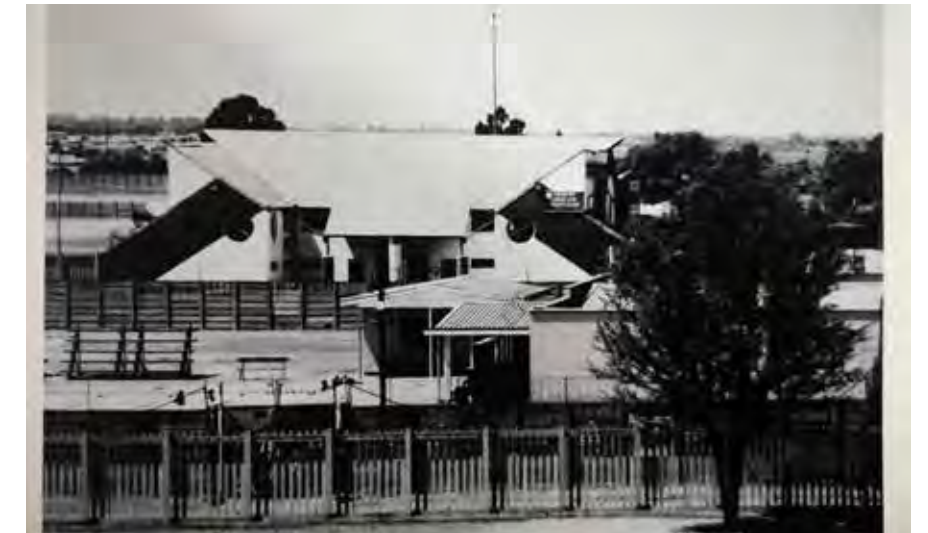
Fig 3.14 - View of Squash courts. (Bhana, 2022)
