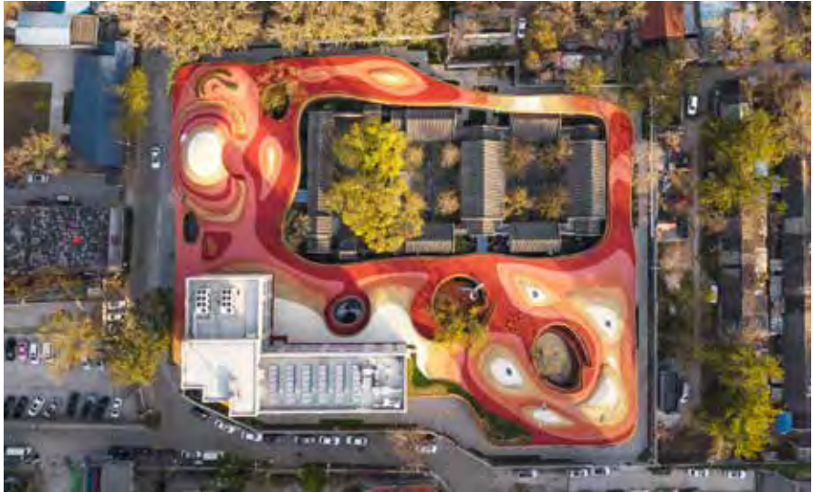
Fig 4.32 - Aerial view of roofscape connecting buildings. ("MAD Tops Beijing Kindergarten with Red Rooftop Playground" 2020)
