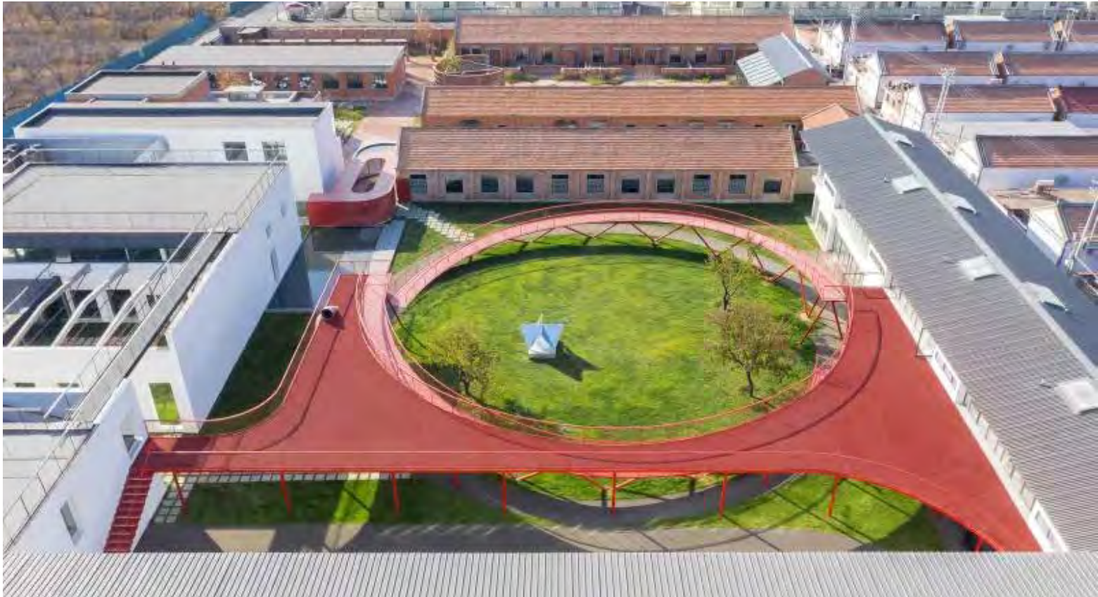
Fig 4.20 - Aerial view of walkway connecting buildings. ("REDe Architects, Moguang Studio, Xia Zhi · The Youth Activity Center" n.d.)
