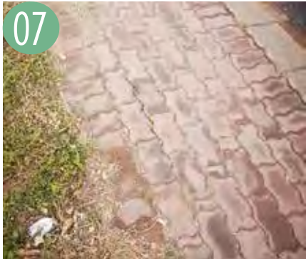
Paving around the edges of the circle.
