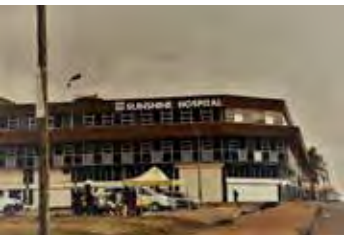
Fig 3.17 - Exterior of Sunshine Hospital. (Author, 2022)
