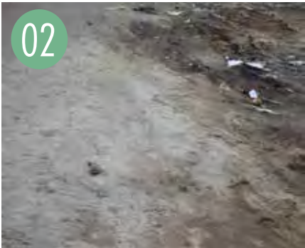
Damp clayey soil.
