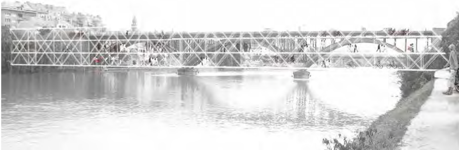
Fig 4.24 - Aerial view of bridge connecting shores. ("José María Sánchez García · Footbridge Across the River Drava River 2012" n.d.)
