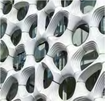
Fig 3.67 - TiO 2 used in facade. ("Mexico City Hospital 'Eats' Pollution: Torre de Especialidades Features Innovate Facade Tiling That Neutralizes Smog" n.d.)
