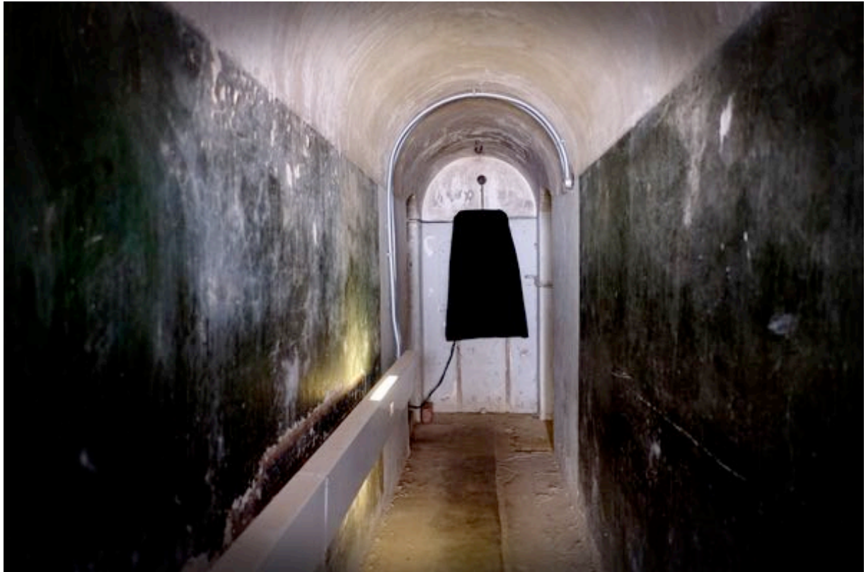
Fig. 8. Room 1 - Entrance Corridor. View from the entrance doorway.
